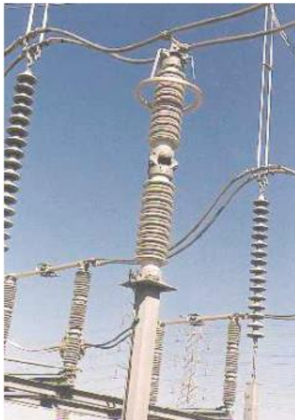
Fig. 26 Lightning arrester.
