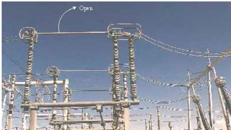
Fig.24 Disconnecting switch.
