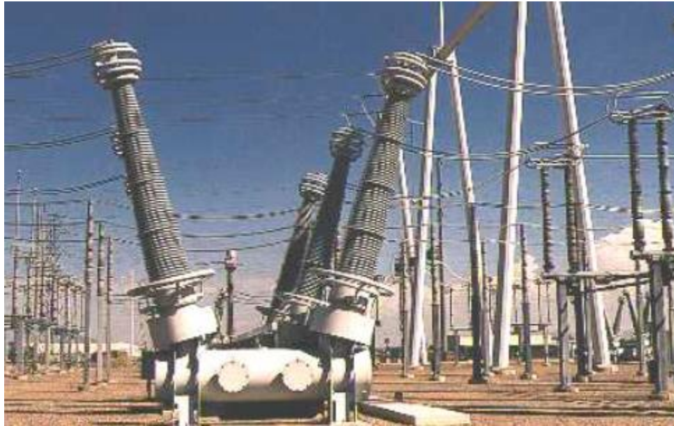
Fig.23 Circuit breaker.
